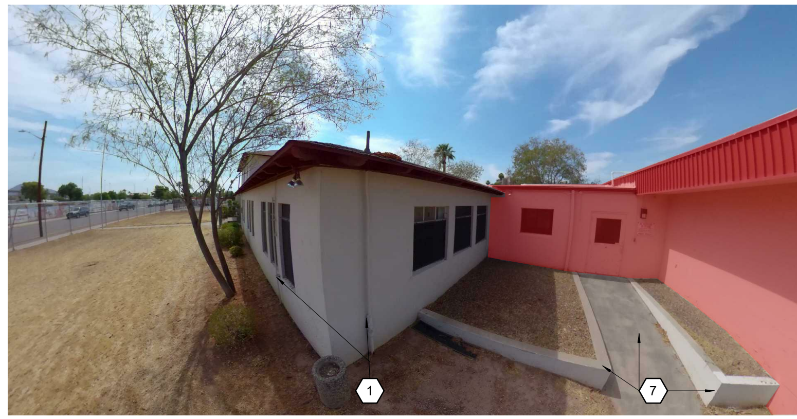
D14 SOUTHWEST EXTERIOR
