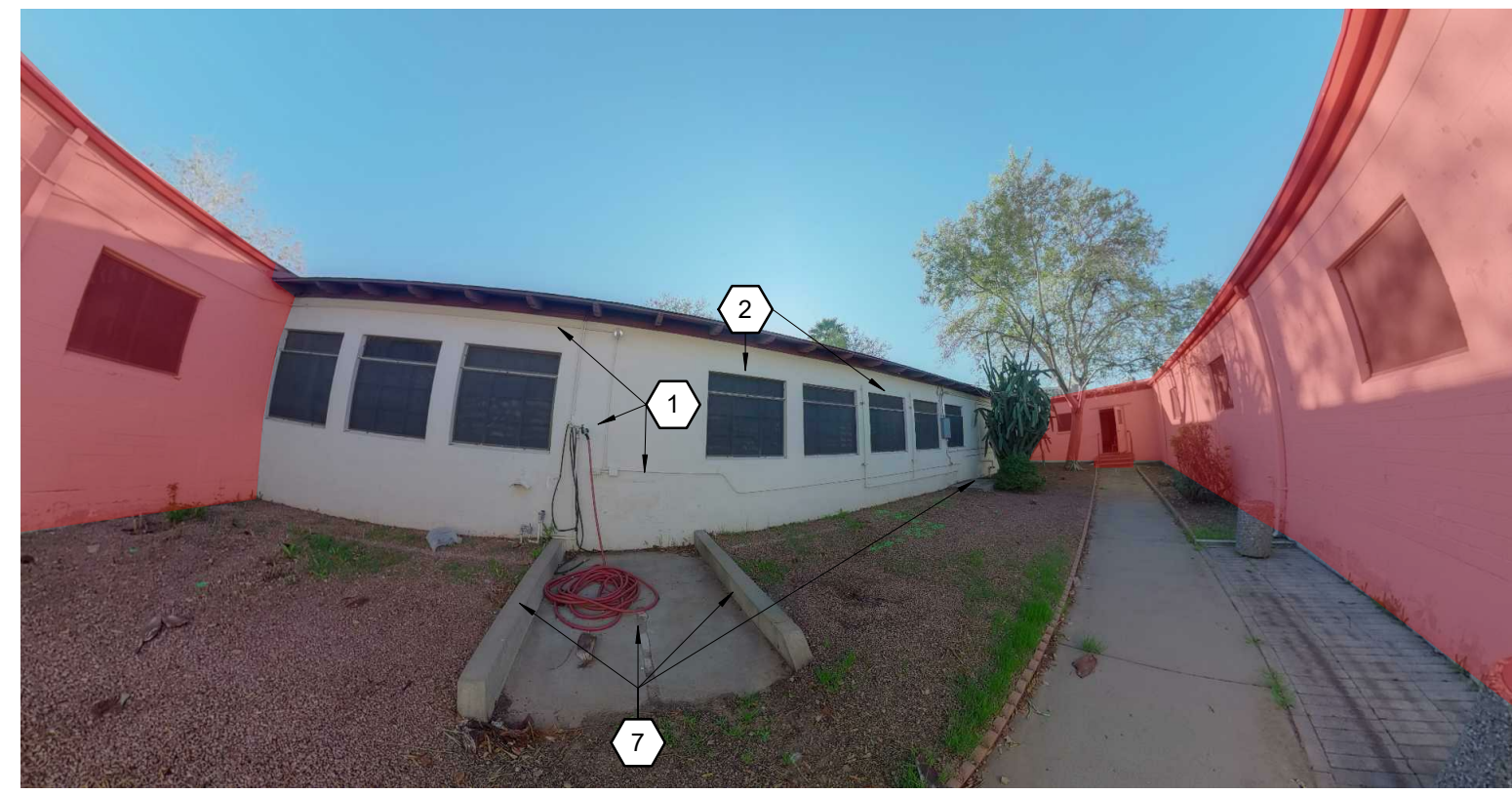
D18 SOUTHWEST EXTERIOR
