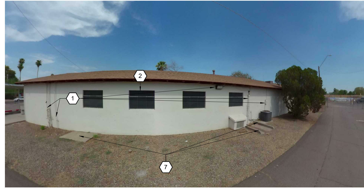
J18 SOUTH EXTERIOR
