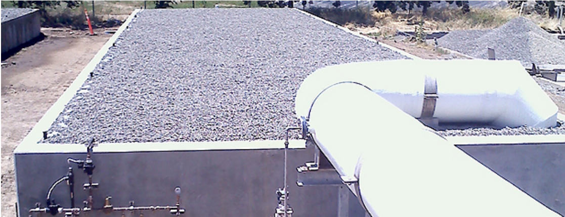
Figure 5-1: Buried Biofilter Example
