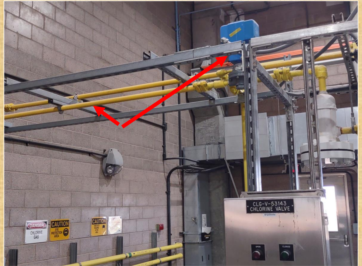
Replace PRV and Chlorine Piping
