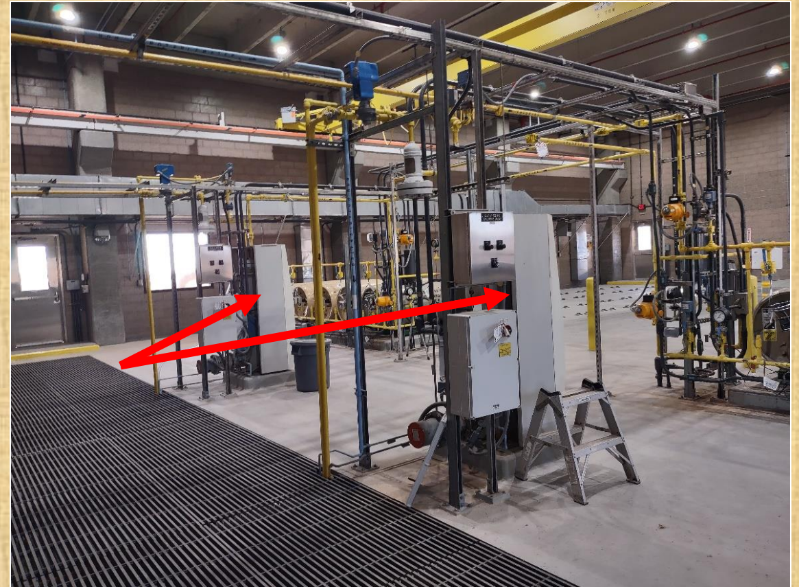
Replace Chlorine Evaporators and Equipment
