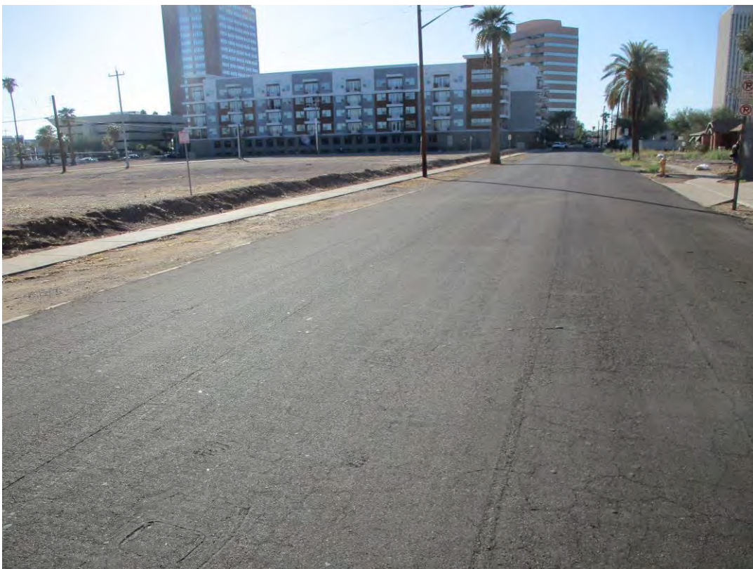
West Along Weldon Avenue, Subject Site at Left
