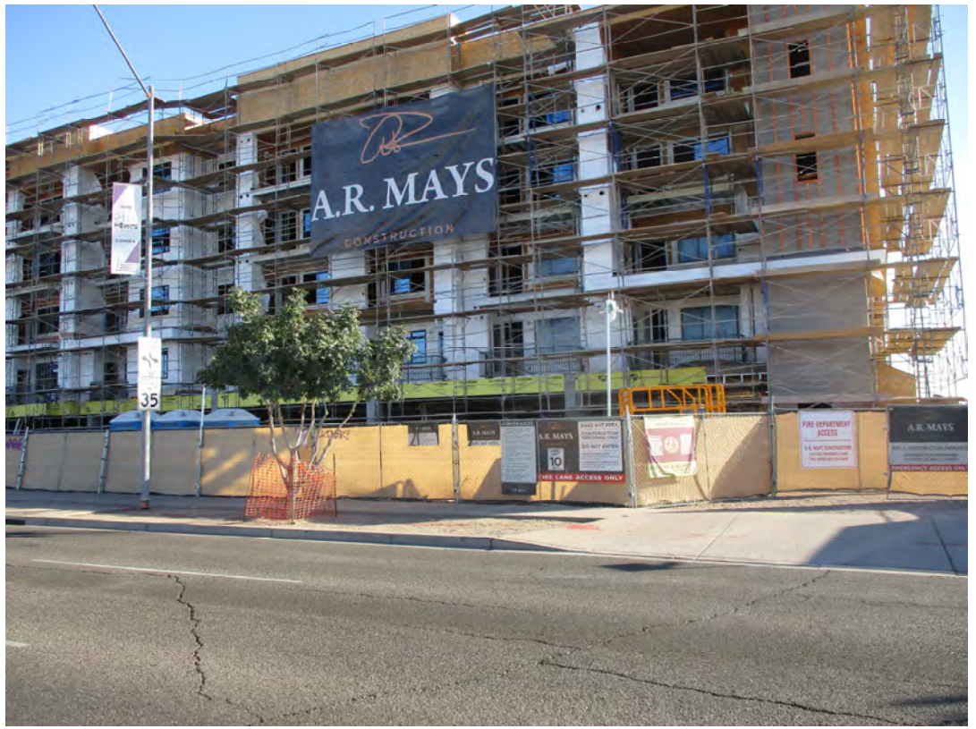
Photograph Of Land Sale 5 (Under Construction)
