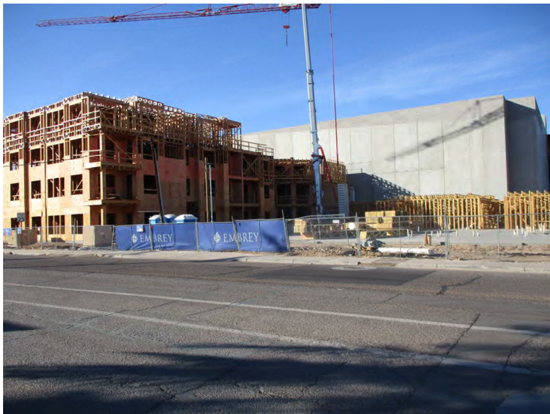
Photograph Of Land Sale 3 (Under Construction)
