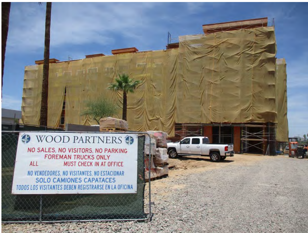
Photograph Of Land Sale 2 (Under Construction)
