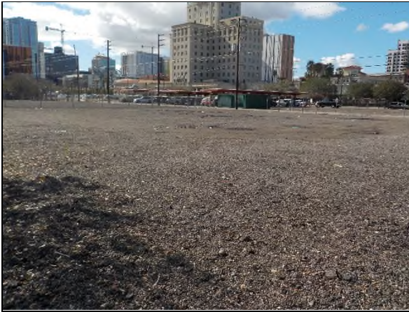
Three Parcels At the SWC Of 1 st And McKinley Streets - View Facing Southwest Across Site
