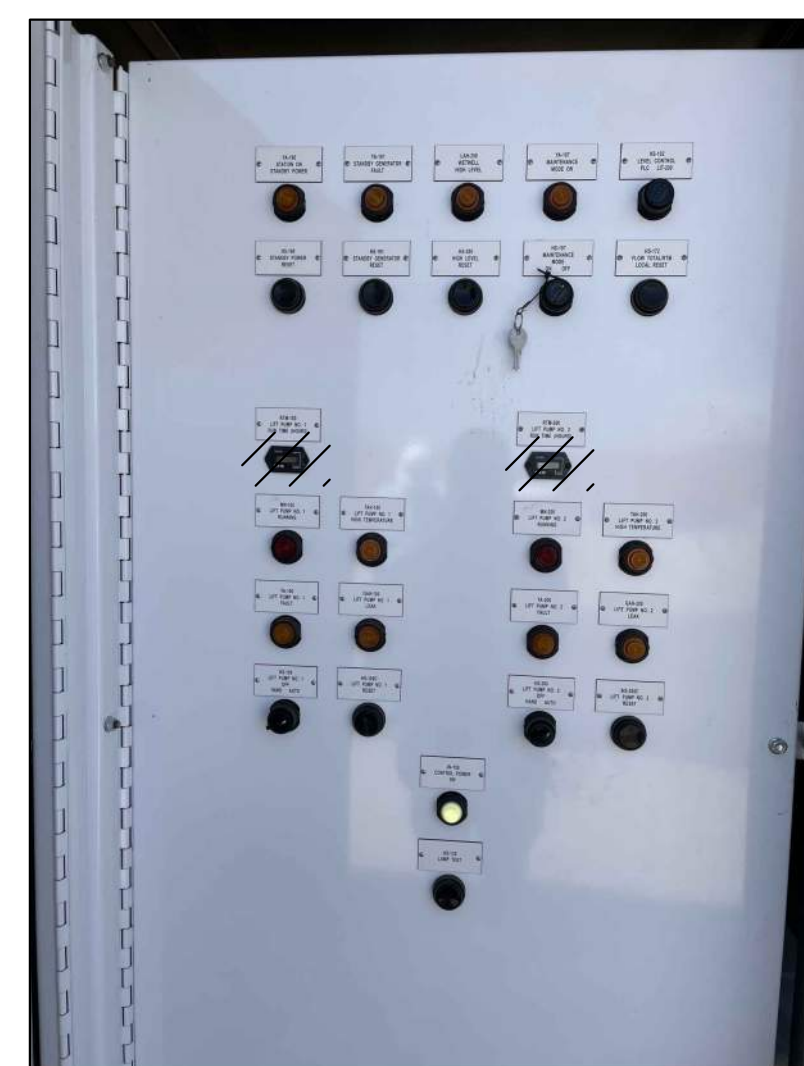
EXISTING LCP-PCP-LS76 LIFT STATION NO.76 PUMP CONTROL SCALE = NOT TO SCALE
