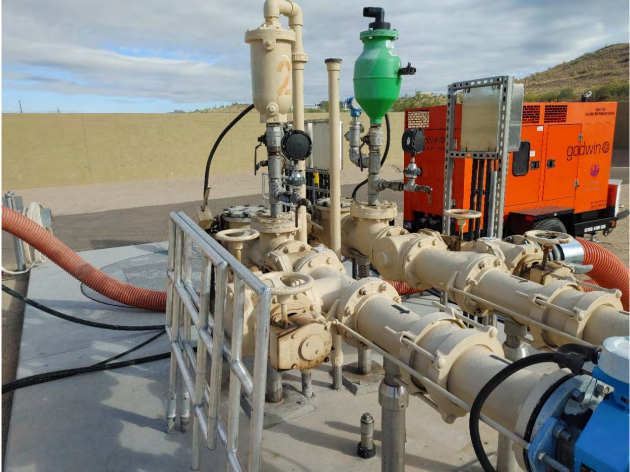
Lift Station 76 Force main piping
