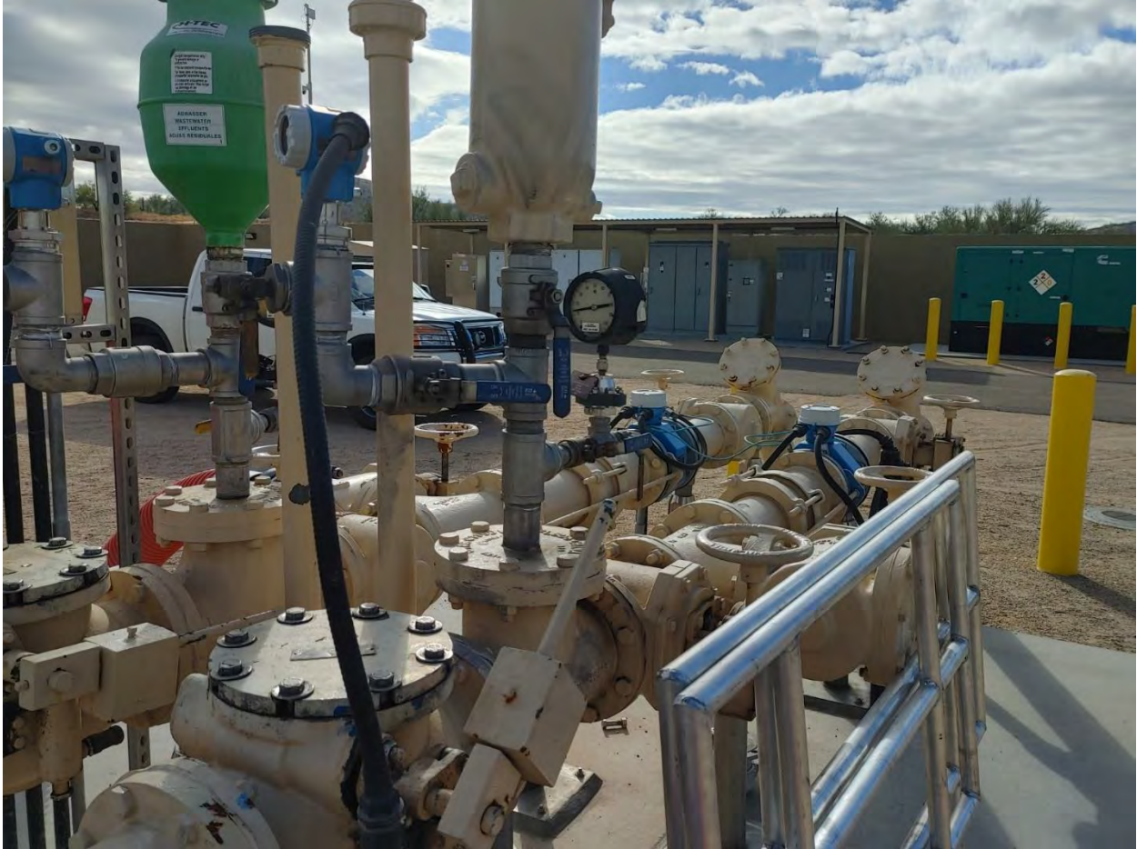
Lift Station 76 Force main piping
