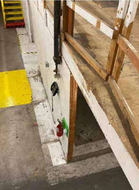
Photos 3 and 4 - Mezzanine Structure
