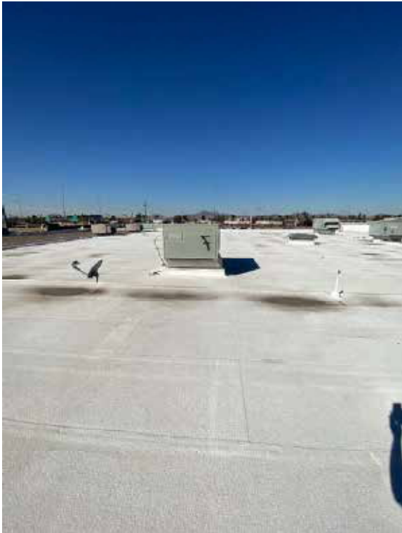
Photo 7 - Existing Rooftop Mechanical
