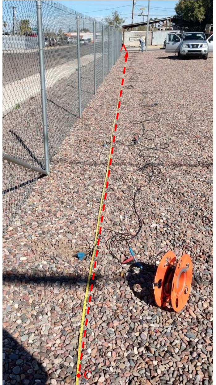
Figure 3; Photo 2: Seismic Survey Line 132A-01 view looking north from Shot Point C toward Shot Point A.
