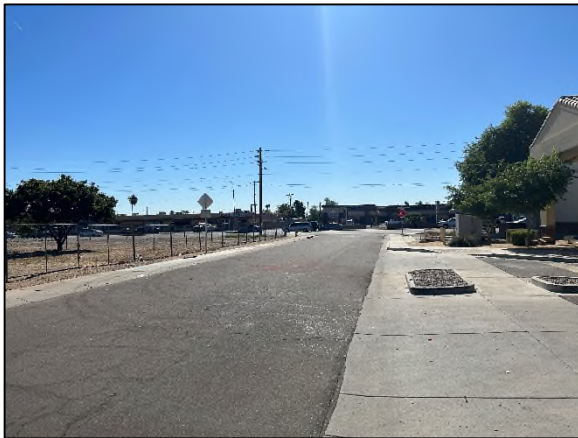
26 th Drive looking south – subject on left
