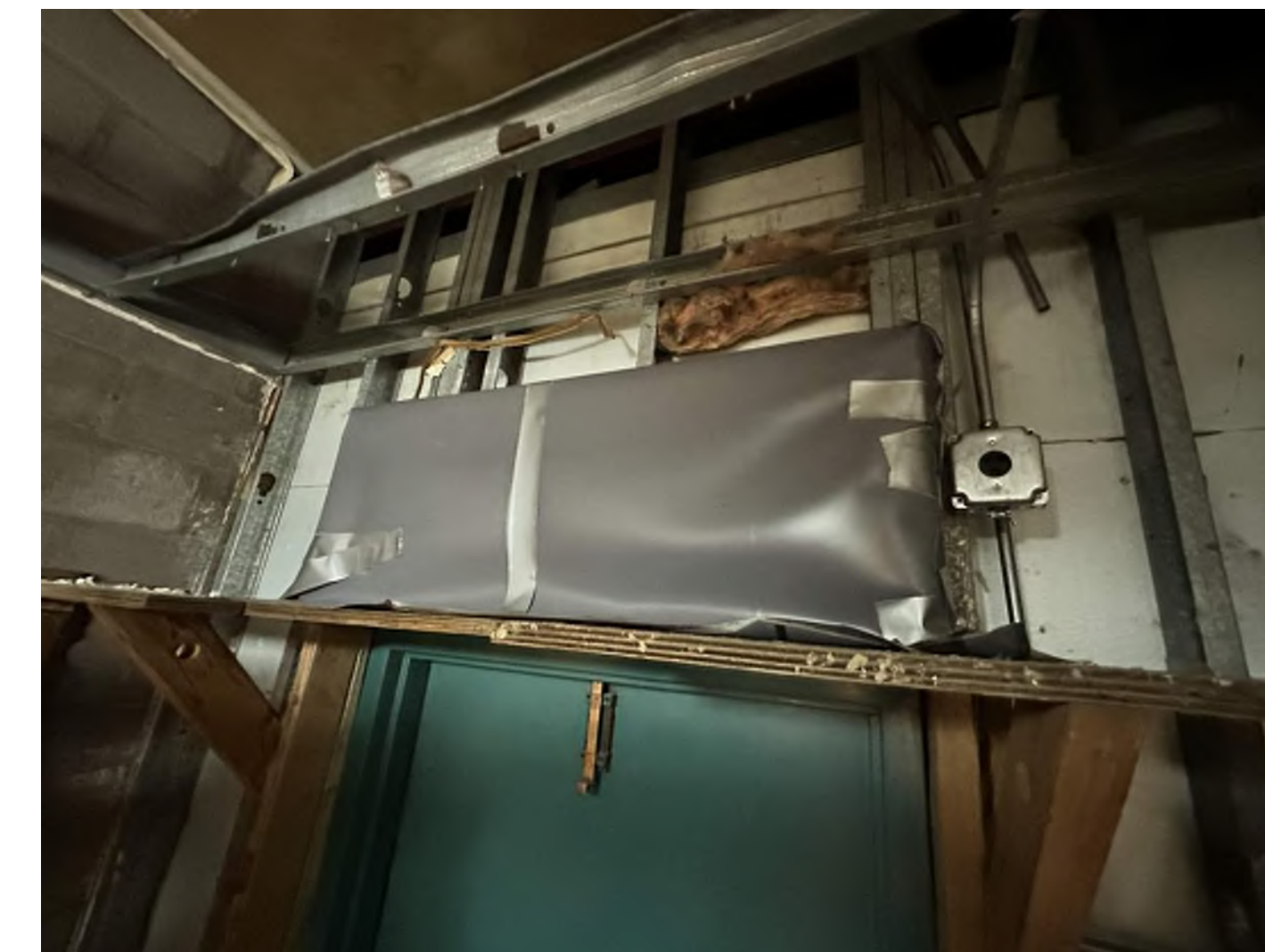
06 VIEW OF BLOCKED OFF DOOR AND VENTILATION (NORTH)
