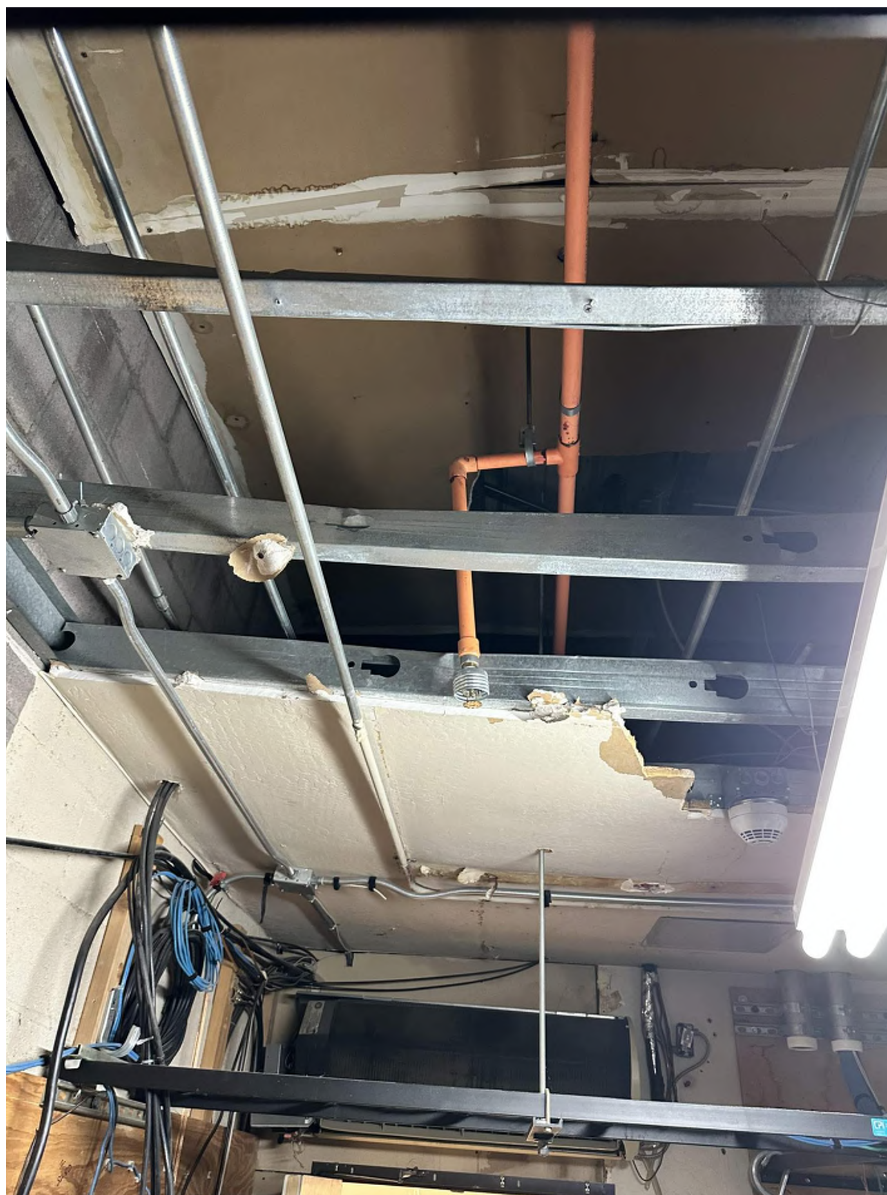
04 VIEW OF IDF ROOM CEILING (LOOKING SOUTH)
