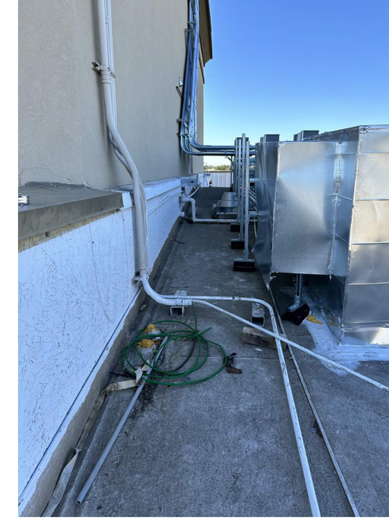
02 VIEW BETWEEN PULL BOXES AND EXTERIOR WALL
