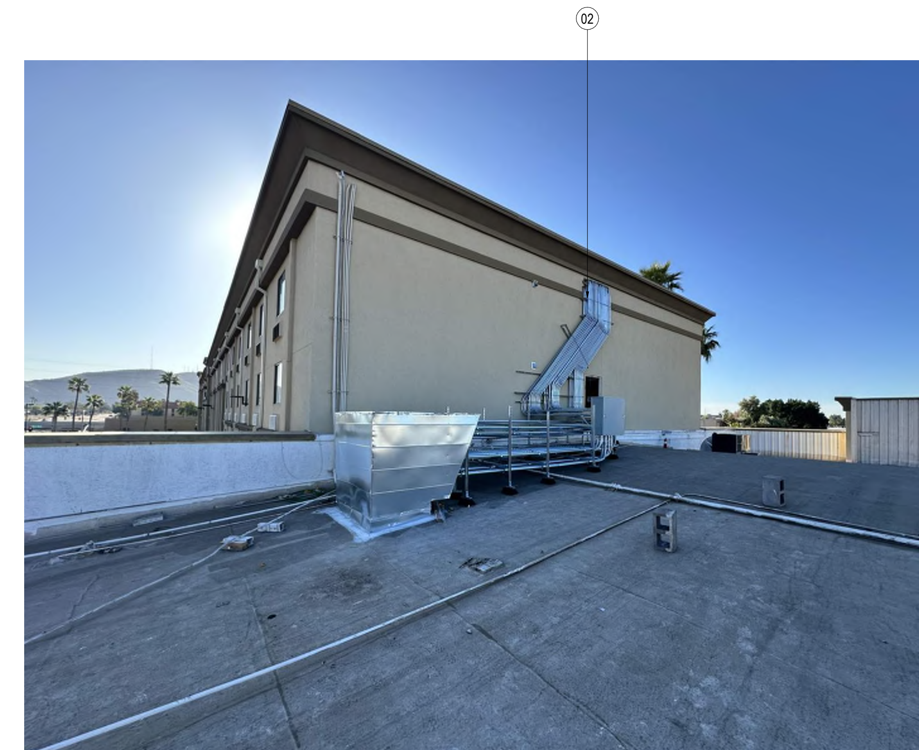
05 VIEW OF EXISTING CONDUITS AND PULL BOXES (LOOKING EAST)
