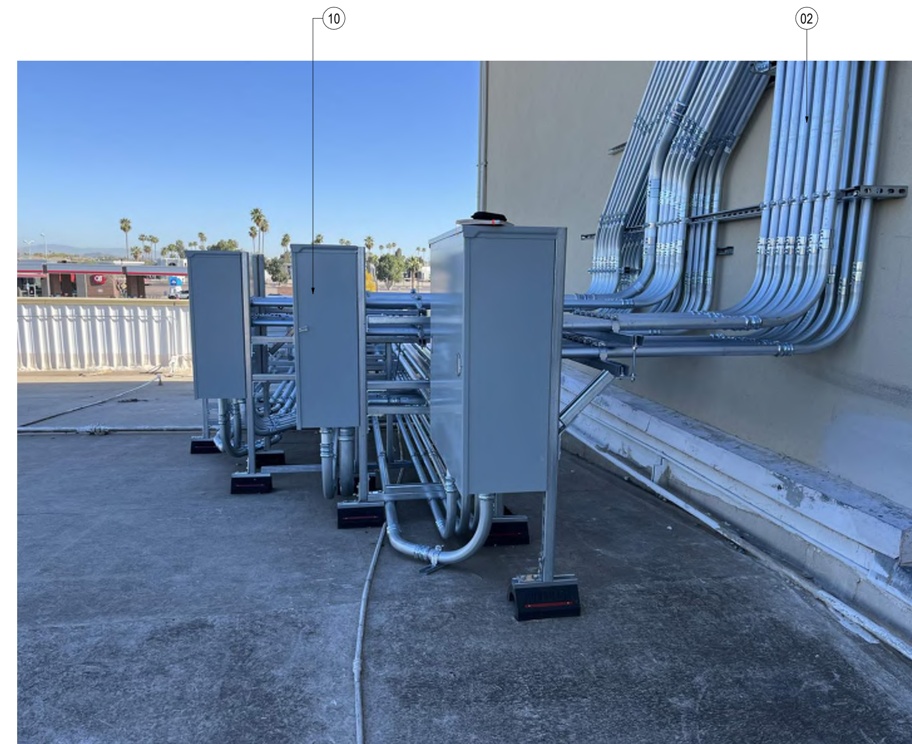
04 DETAILED VIEW OF EXISTING CONDUITS AND PULL BOXES
