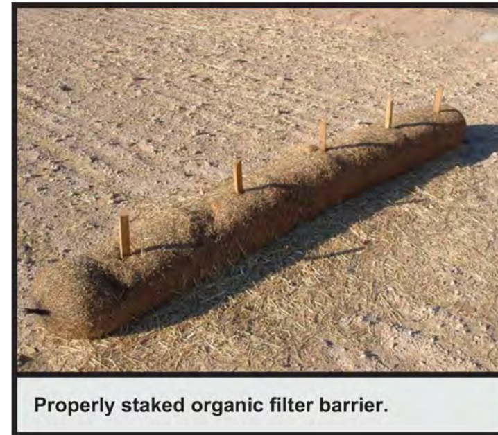
Properly staked organic filter barrier.
