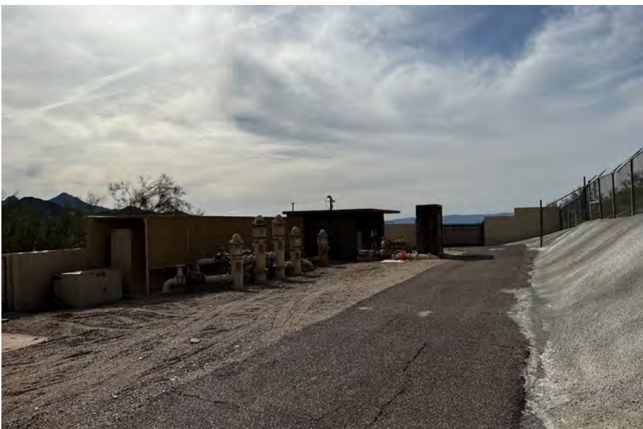
City of Phoenix Well Site
