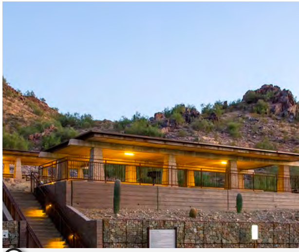
8 Refurbish Existing Ramada
