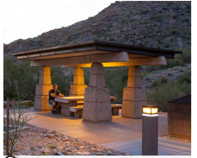
9 Refurbish Existing Ramada
