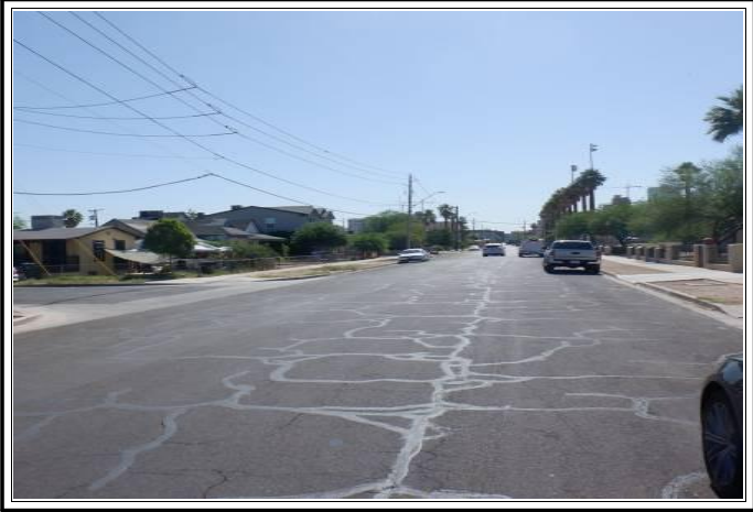
Additional street scene
