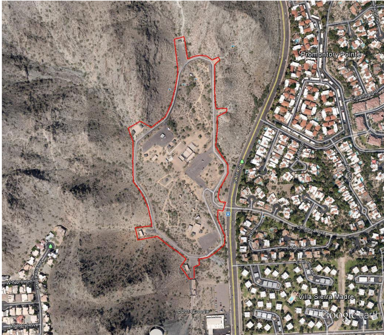
North Mountain Park Aerial Photo
