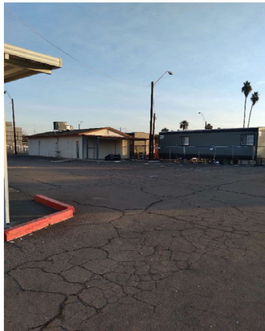
Picture 2 - Central area of the site, facing northeast.
