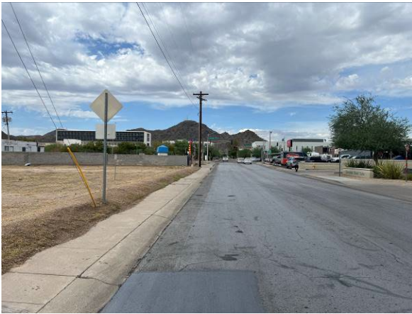
Looking north along 3 rd Street
